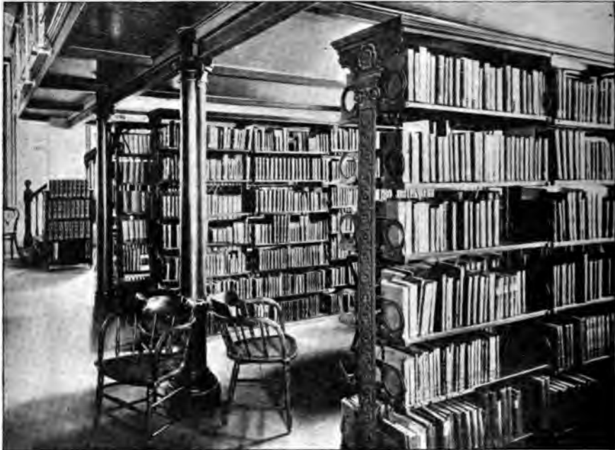
STEEL SHELVING SUPPLIED TO THE PUBLIC LIBRARY OF QUEENSLAND, Brisbane.
